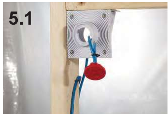
Figure 5.1 & 5.2: Make a loop with your prewire and run it through the RDM threaded insert opening, then wire tie the loop to the back of the RED mud shield. Insert the RED mud shield into the RDM threaded insert, and turn clockwise to lock in place. You may need to hold the threaded insert to keep it from spinning. You are now ready to install the wall finish.
