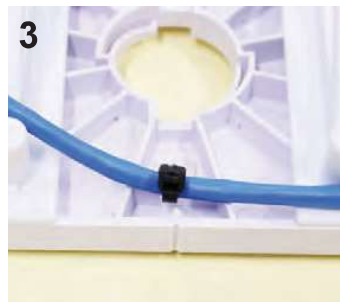
Figure 3: With your location selected and wiring ran, use a wire tie (not included) to fasten the prewire to the rear of the RDM platform. Leave excess cable to be pulled through the RDM insert opening. This will ensure that your prewire does not get damaged or go missing during the other construction stages.
