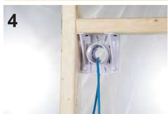
Figure 4: Mount the RDM to the two-by-four, either vertically or horizontally, using two wood screws (not included). Double check to make sure that the mount is flush and plumb with the wall/studs. If the mount is set back slightly from the stud, that is better than sticking out too far out. Having the mount sticking out too far will affect the wall finish install. You can then install the threaded insert by screwing it into the front or back of the RDM mount. Turning clockwise from the front or back.
